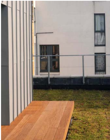
Sedum roof Green feature of the previous HCPC project at 22-26 Stannary Street
