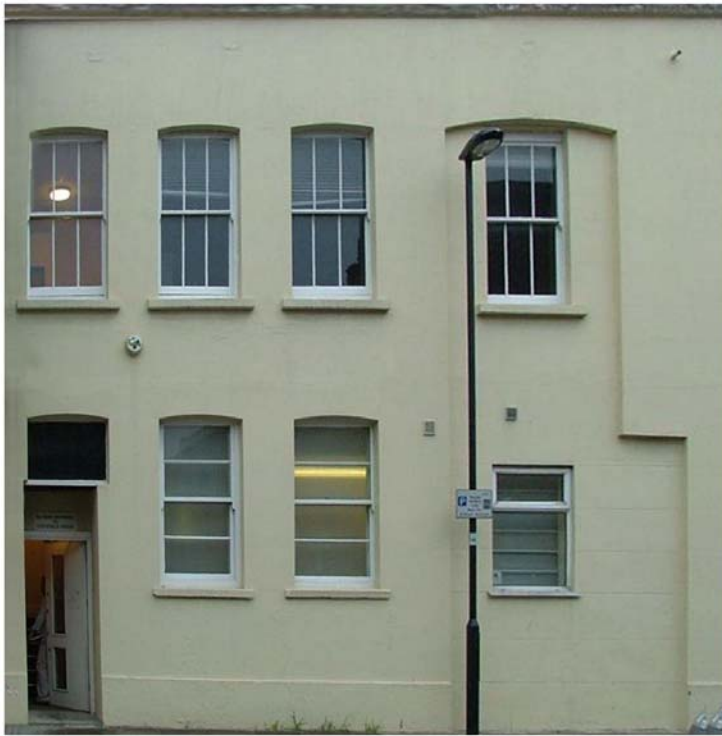
Photograph of existing facade of 18a Stannary Street, with double height opening on right
