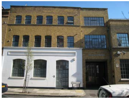
Whitacre Mews street facade , Stannary Street
